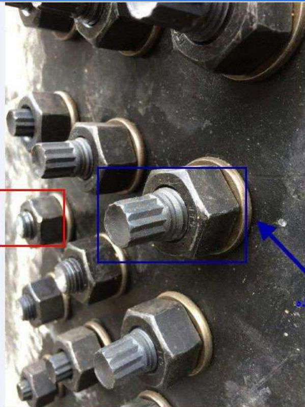
Tension Control Bolt (TC Bolt)
