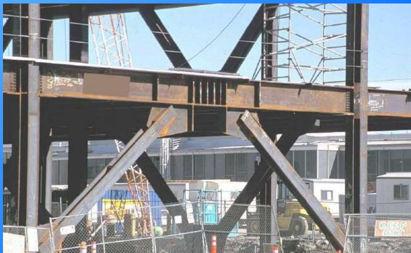
Figure 25 Different types of eccentric bracing
